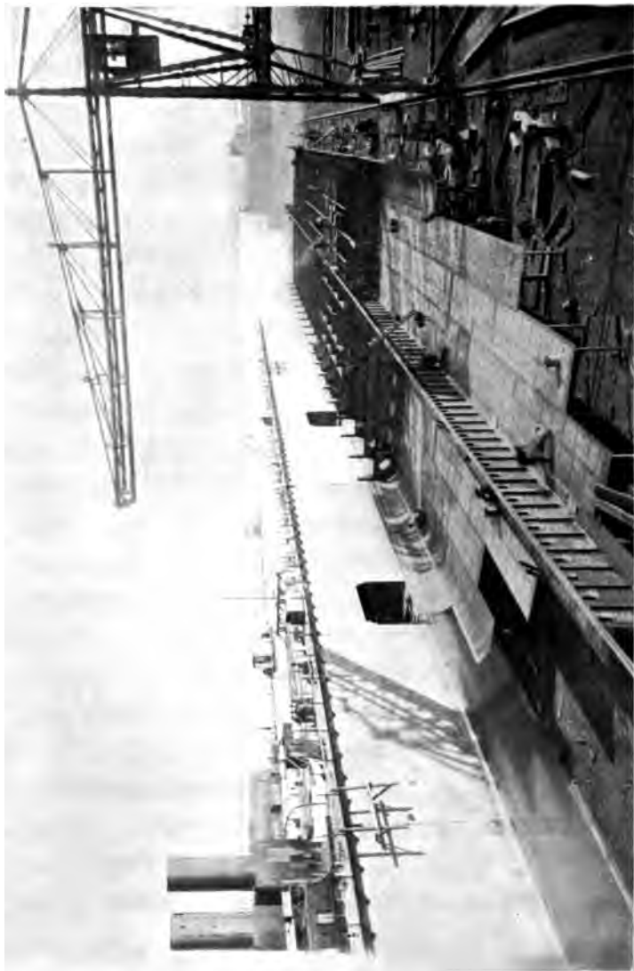
Second Step—Laying the Keel, or Bottom of the Ship, on the “Keel Blocks.”
